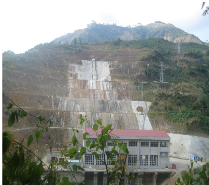
Fig.1: The Xekaman 3 hydro power plant
