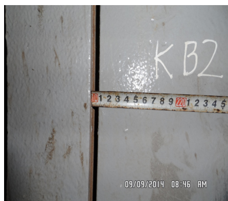
Fig.10. The compensator at the horizontal penstock
